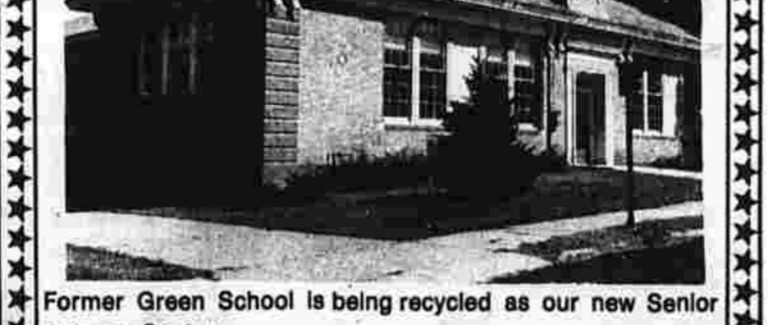
Former Green School is being recycled as our new Senior Citizens Center.
